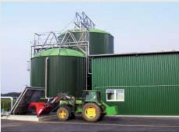
Feedstock mixing bin, buffer tank and fermenter
